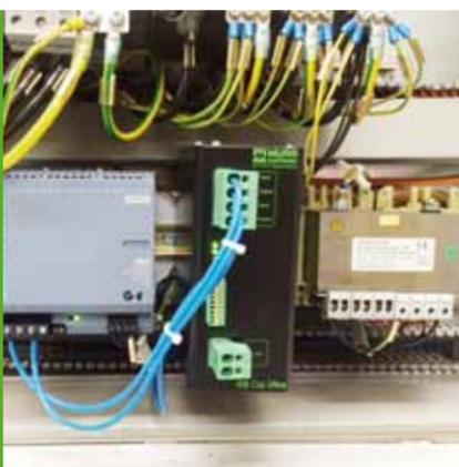
The power grid at the manufacturing facility often has voltage fluctuations. In the past, this caused a CNC lathe control, which is part of the production line, to fail. As a result, the PLC lost its data and production stopped. It would take almost an hour and a half to get the lathe running again and it took as much as ten hours to restart the complete production line. As you can see, the mains' fluctuations and resulting system outages increased costs dramatically.
